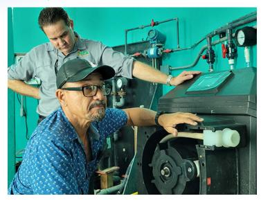
The facility had been using four FLEXFLO M4 Peristaltic Metering Pumps to dose polymer to the system, however, when they learned of the larger capacity FLEXFLO M5 pump they felt it would be advantageous to make the switch to one M5 running at 33% capacity. A second M5 was purchased as a backup pump.
